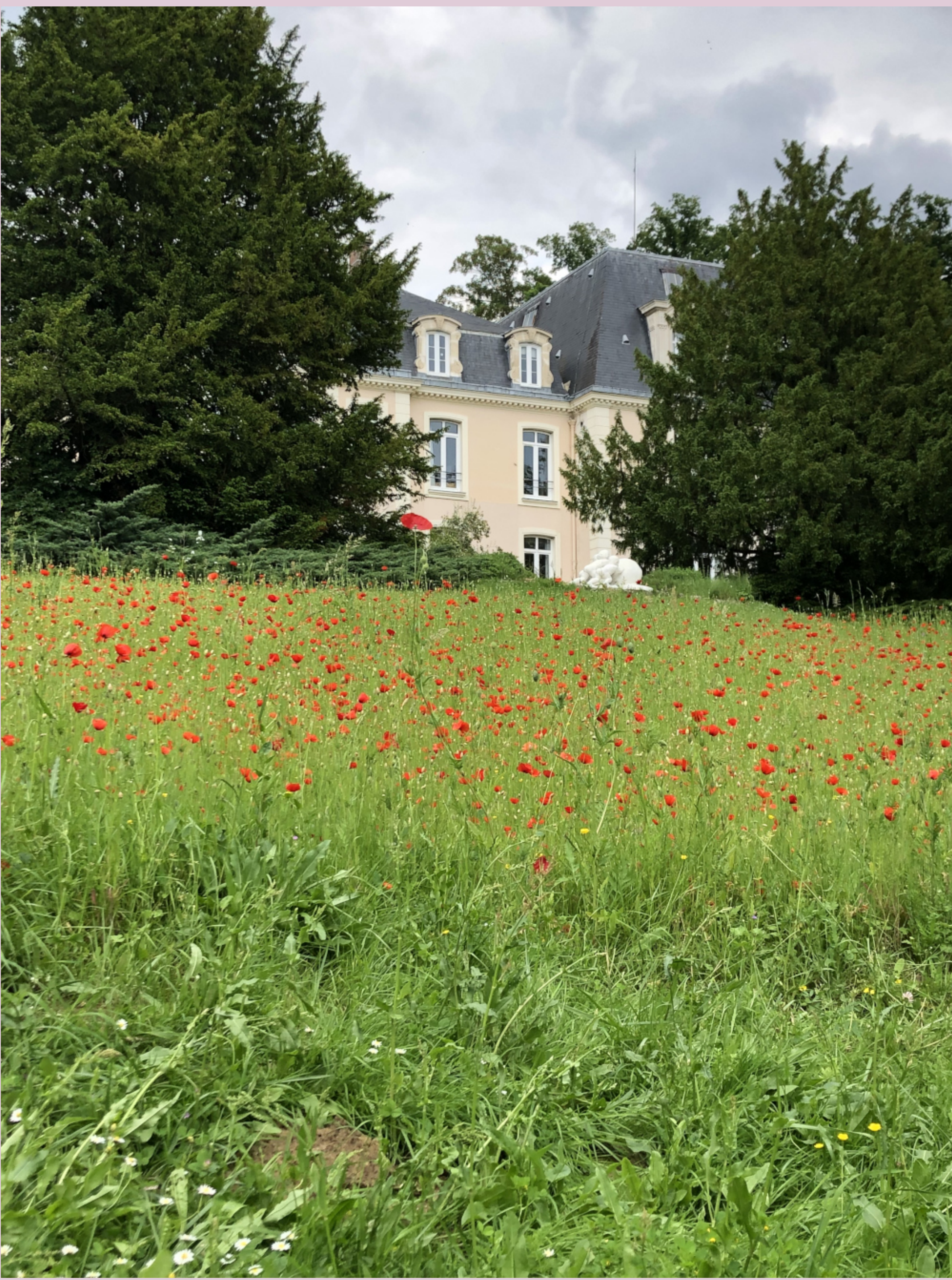
Figure: Vue of building 300, aka "le chateau"
